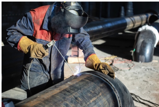
Figure 5.3: Welding Application with Basic Electrode
