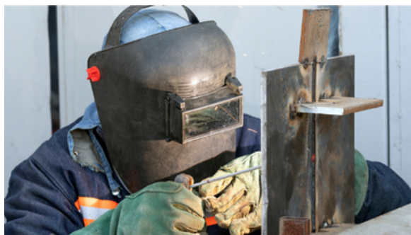
Figure 3.2: Vertical Welding with Electric Arc
